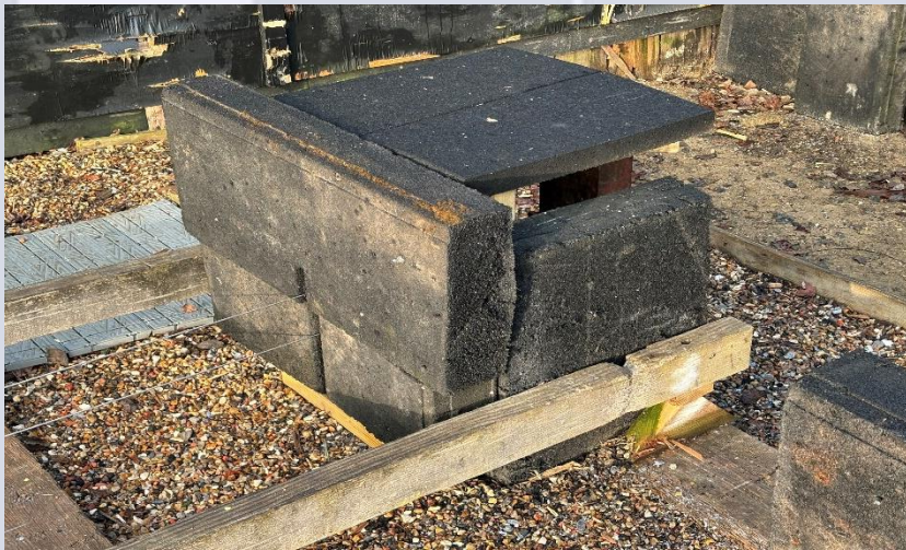
Rebuild and modification to the Cable return Housings
