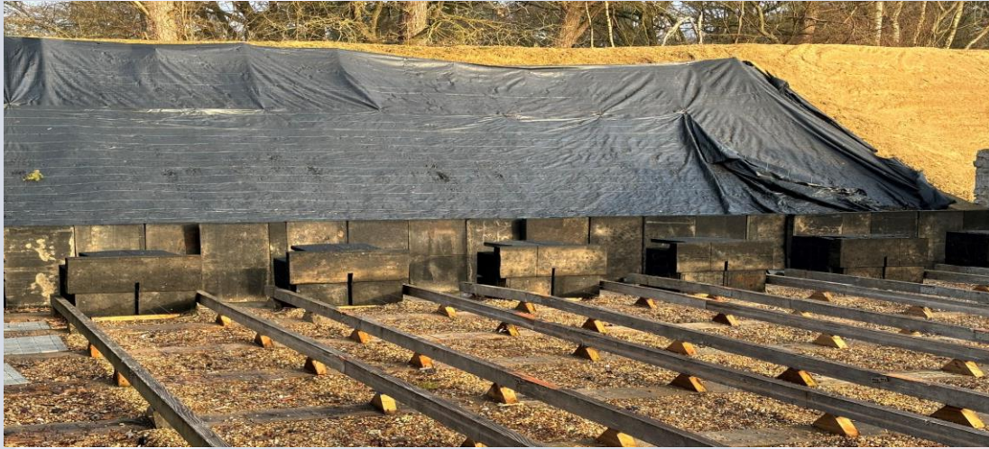
Structural repairs to the running track
